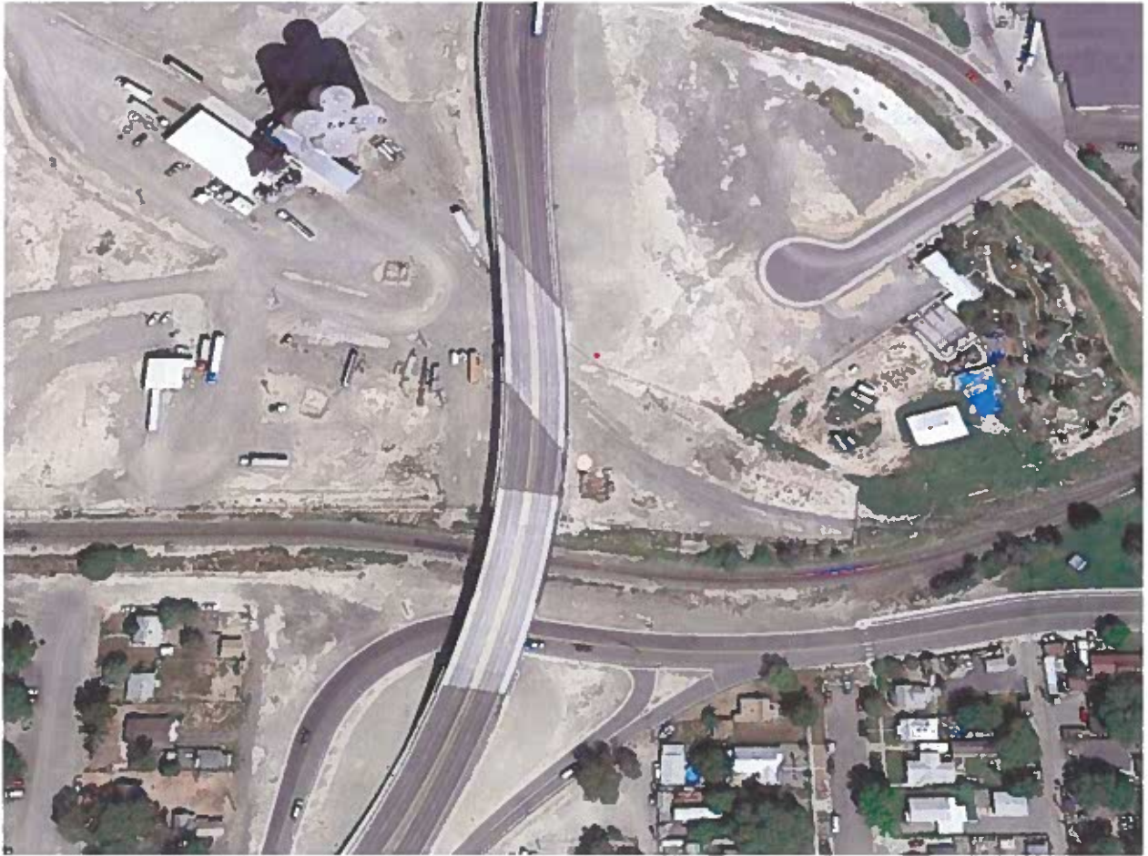
* Bridge over 1st Street and Union Pacific Railroad
