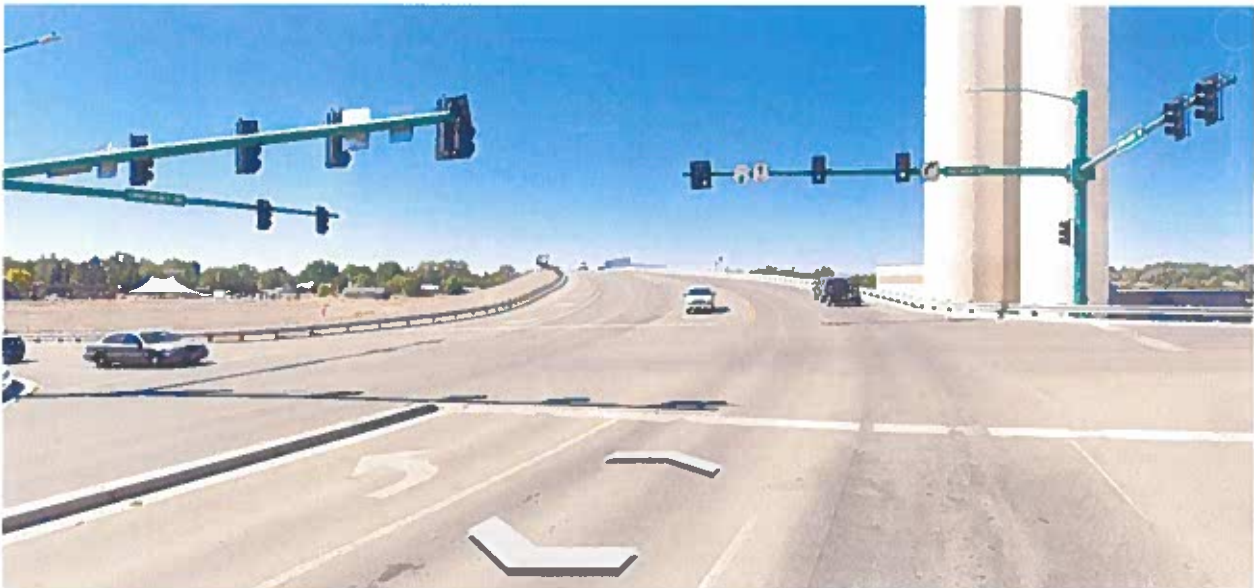
* Intersection/ Traffic Signal at Palmer Street and Confluence Drive
